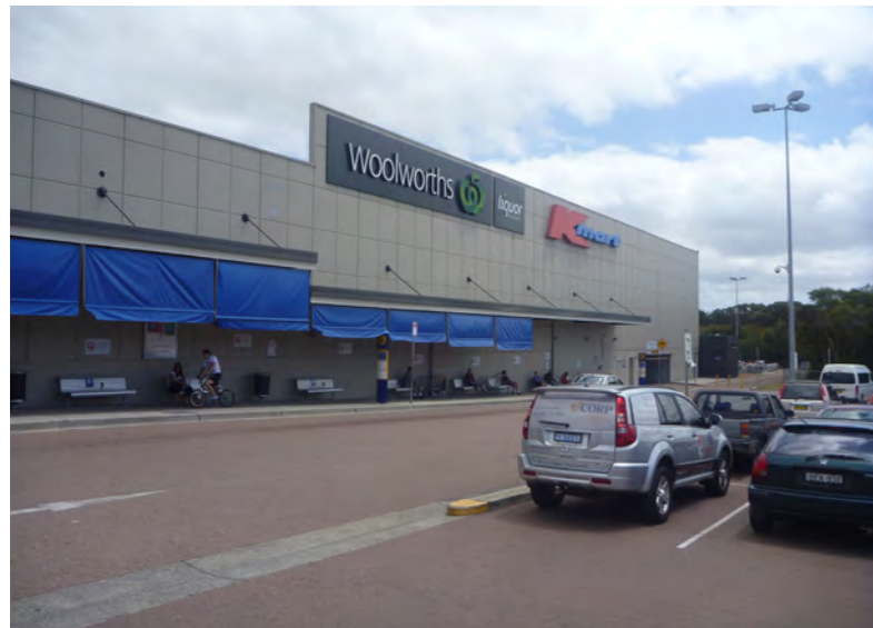
View of existing bus interchange.
