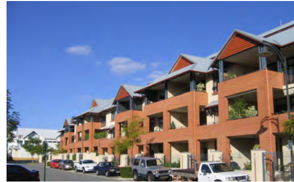
Built form that addresses the street.
