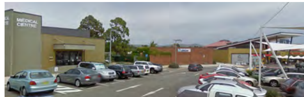
Existing street view of site.
