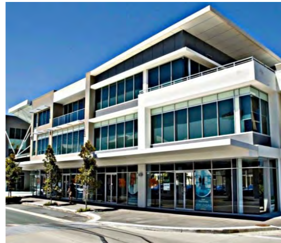
An example of low rise office building.
