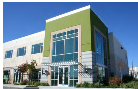
An example of low rise office building.
